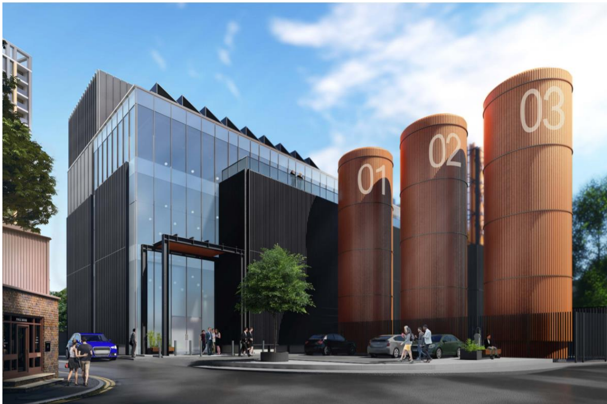
The Energy Centre scheme under construction (granted Planning consent 22 March 2019)
